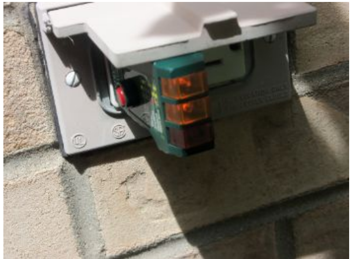
Outside GFCI operates.
