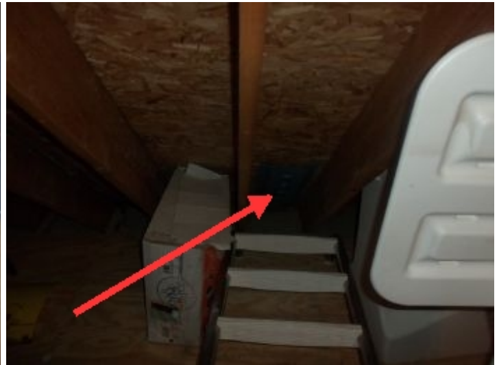
Proper venting installation , Baffles installed.
