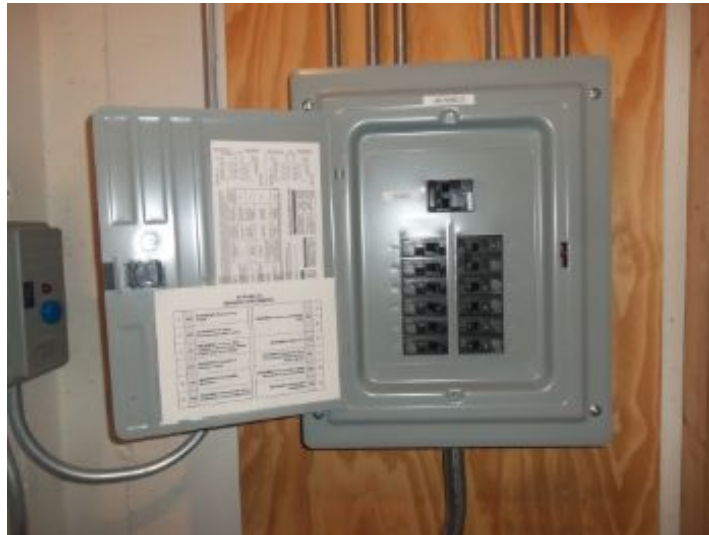
100 amp sub panel, all breakers labeled
