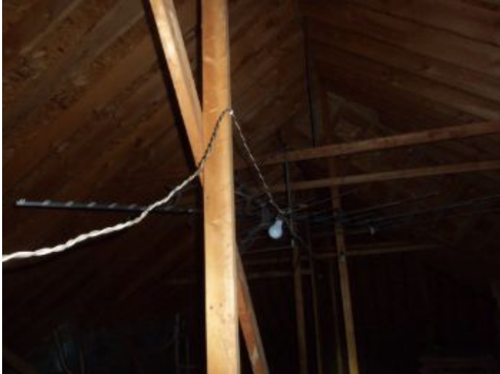
120 v exposed wire, recommend removing.
