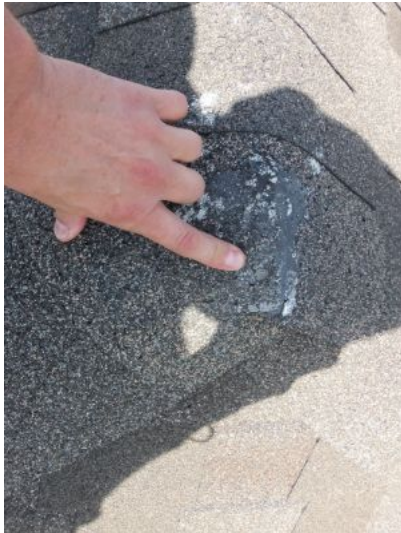
exposed roof nails
