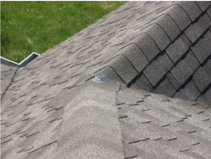
exposed roof nails
