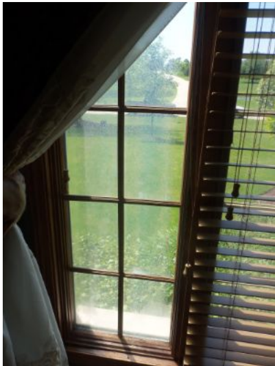
Office, main floor, window seal cracked, recommend repairing or replacing.
