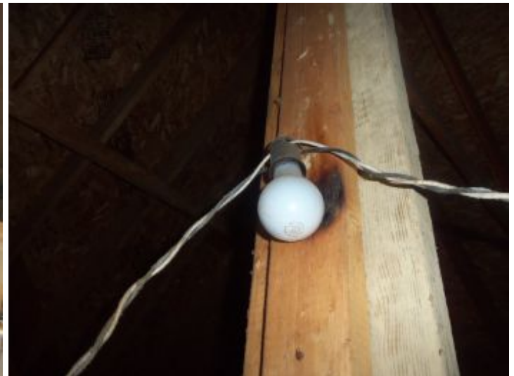
Incaadesant bulb creating a fire hazard, recommend removing or installing a globe.
