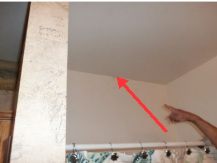
Evidence of water damage in the bathroom ceiling, recommend asking seller for an explanation.
