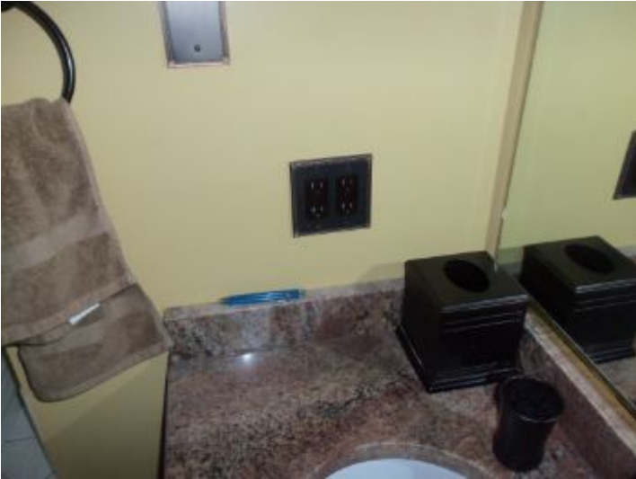
Missing GFCI in Master Bathroom.
