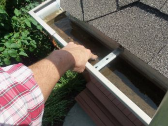
Standing water on NE gutters, due to clogged strainer.
