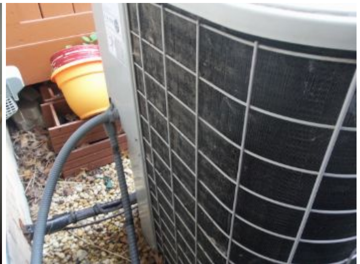
Cleaning required on the back side of the Air Conditioner.
