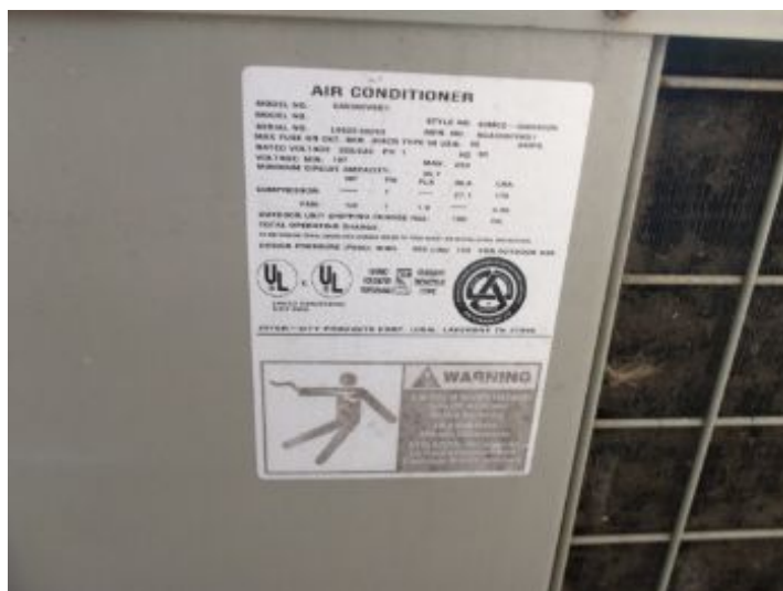
Air condenser, Manufactured in 1996, units operates as designed.
