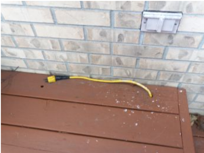
Possible tripping safety hazard. unknown where this leads to?
