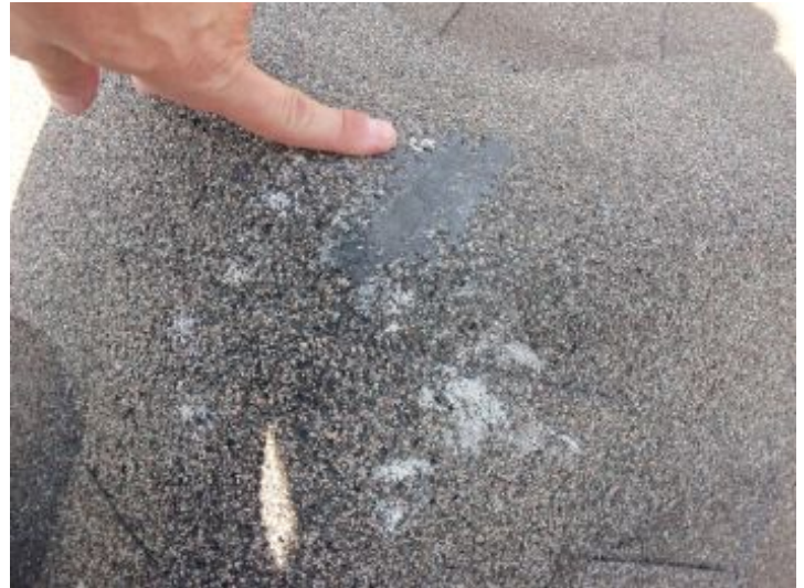
exposed roof nails
