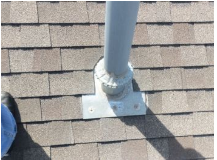
Flashing around Vent is satisfactory.
