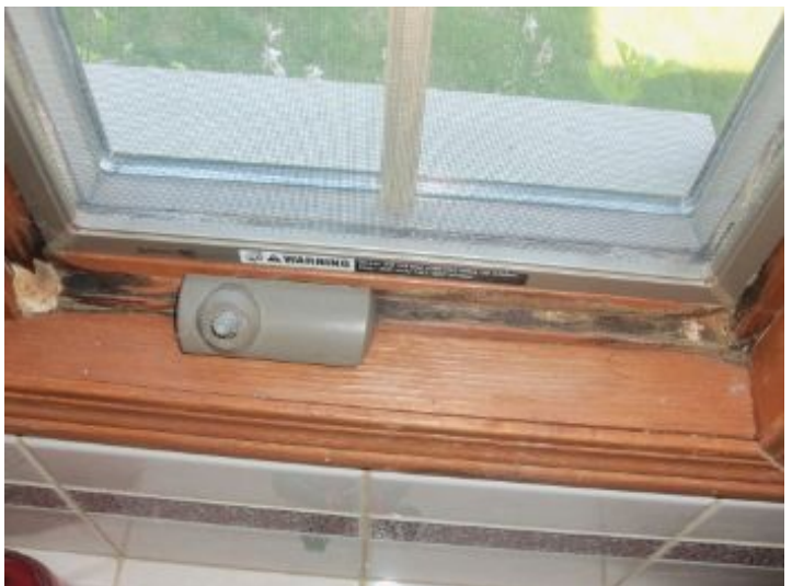
Master Bathroom, evidence of water / moisture on the window.
