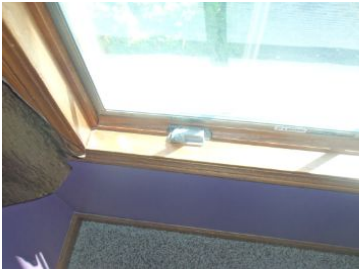
missing crank handles throughout the home.
