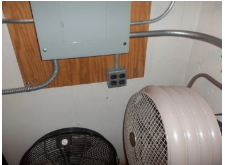
Missing GFCI in the Basement
