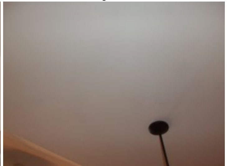
Evidence of possible water damage, front entrance ceiling, recommend asking seller for an explanation.
