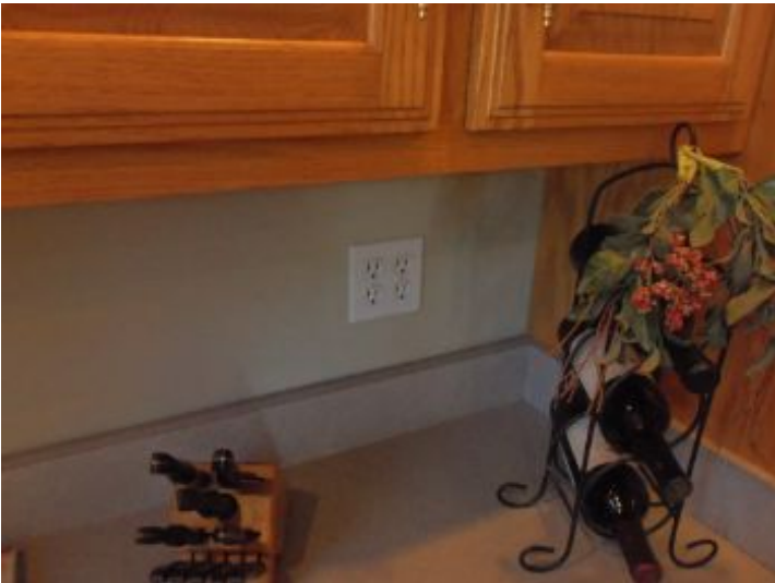
Kitchen, No GFCI present, recommend replacing all outlets with GFCI.
