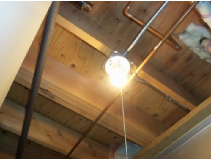
Missing Globes in the basements closets.
