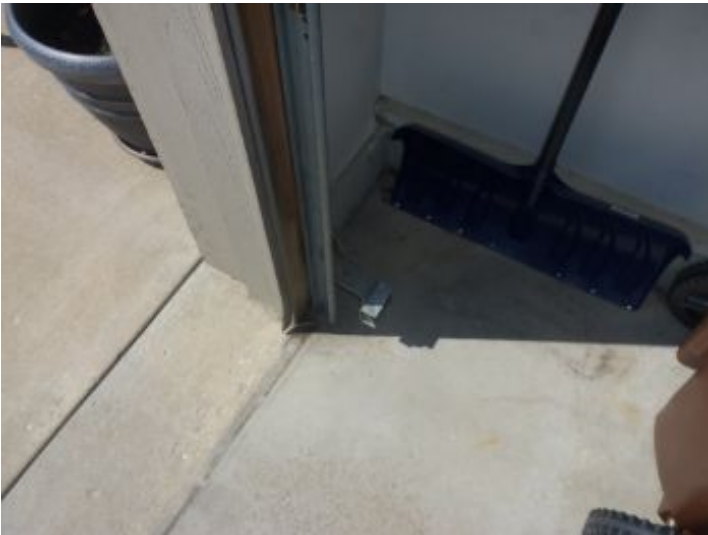
Garage photo eye properly functioning.
