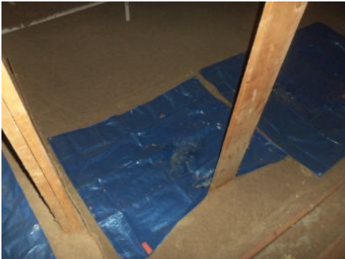
Tarps in the attic? recommend asking seller for an explanation.
