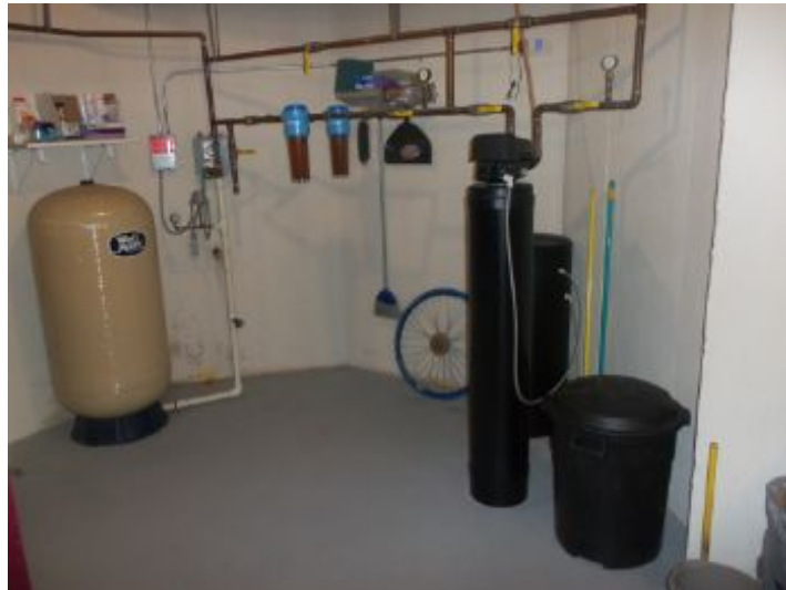
Water Softner System, observed to be piped correctly.
