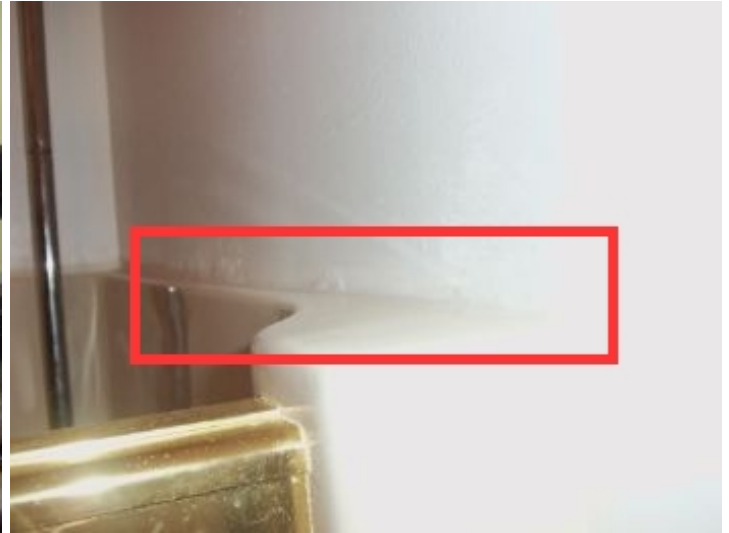
Master Bathroom / Shower, evidence of water damage to walls.
