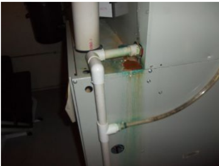
Condensate leaking from the furnace, recommend repairs.
