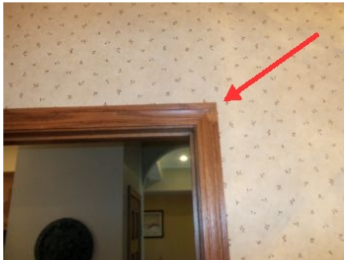
Damage to restroom trim.
