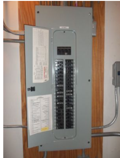
200 campo service, located in the basement. All breakers labeled
