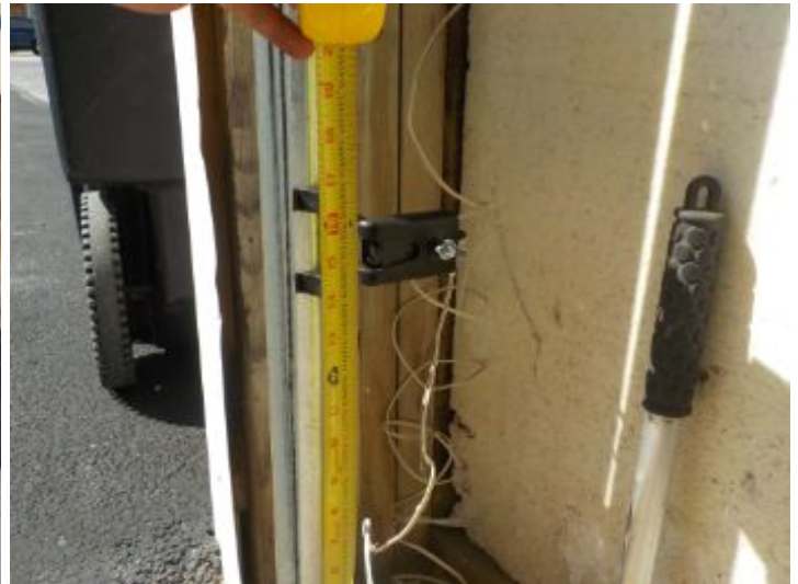
Garage door eye should be installed between 4"-6" from the slab.
