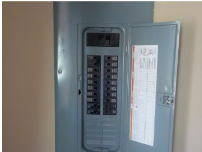
200 amp panel, located in the BD #1, not all breakers labeled
