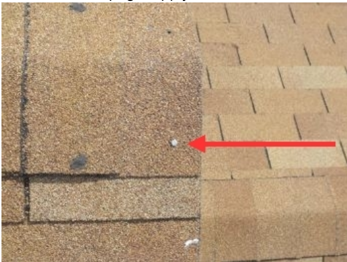
Exposed surface nails on roof vents should be covered with a sealant to ensure against water seepage, apply as needed
