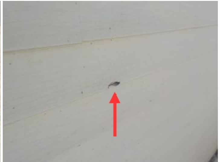
Garage, damage to the siding, may lead to moisture intrusion
