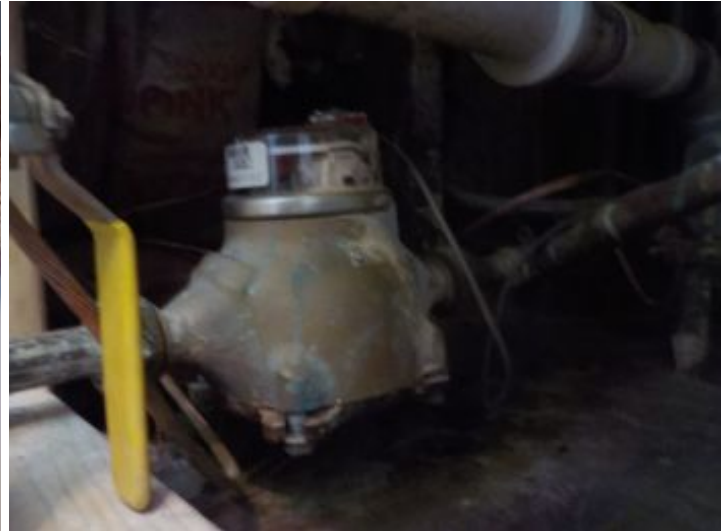
Water meter located in access panel inside laundry room, limited view.
