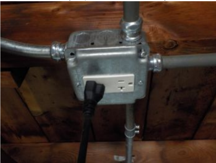
Garage, install a GFCI
