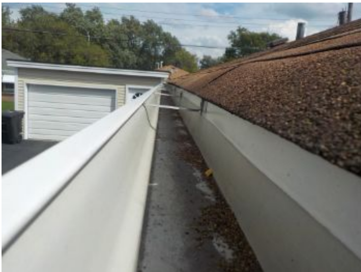
some granule loss in the gutters.
