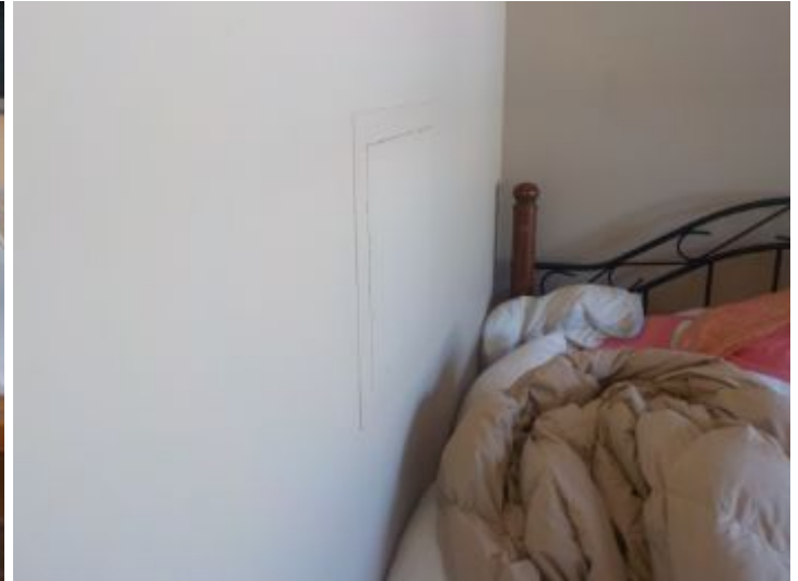
Access panel for the bathroom, unable to access due to personal items.
