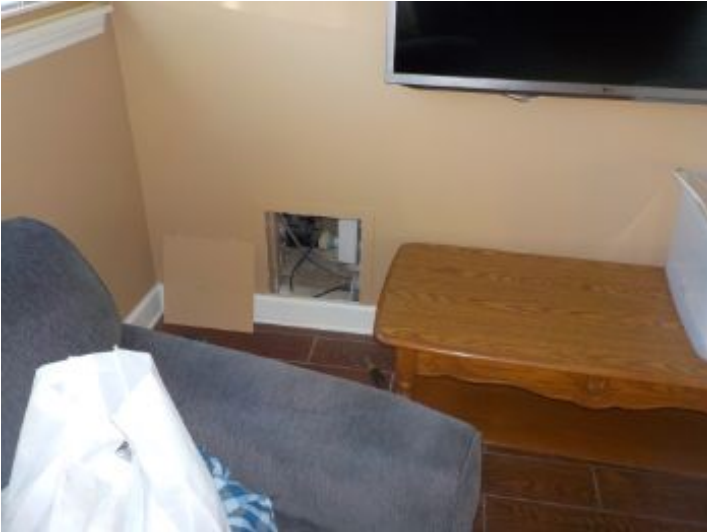
Access panel located in the living room, Pump for the tub.
