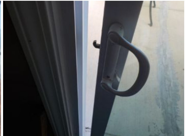
Bedroom door does not secure properly, recommend repairs.
