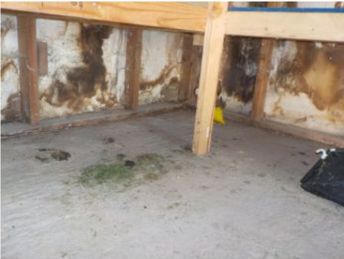
Garage, Evidence of moisture
