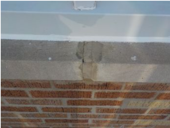
Hairline crack in window sill, recommend repairs to prevent water intrusion.
