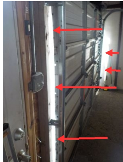
Garage door, should be butted up to the wall. Water, moisture, wind, snow, rodents can enter the garage.
