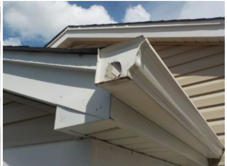
Front Canopy, No Gutters.
