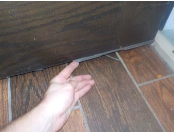
front door, weather stripping damaged.
