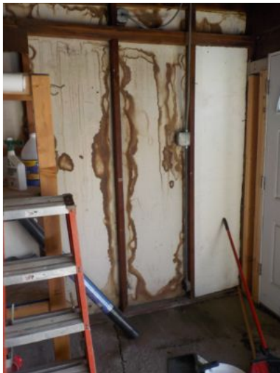
Garage, Evidence of moisture
