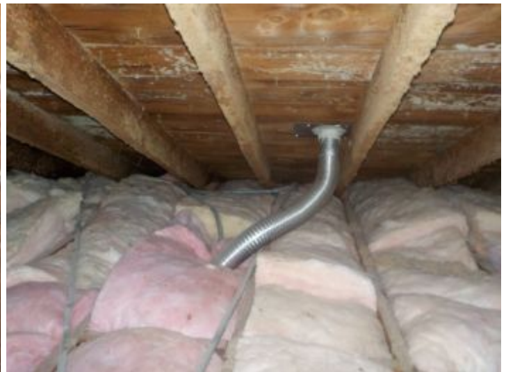
Attic insulation satisfactory
