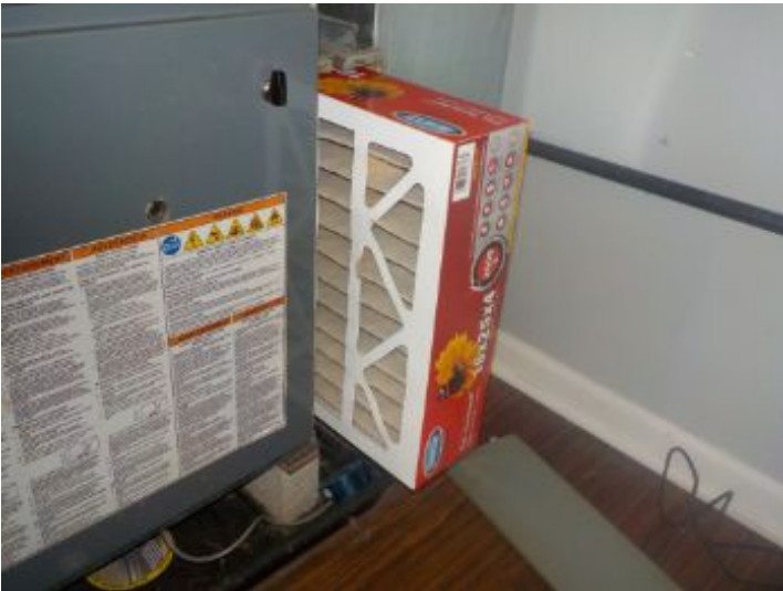
Firnace Filter, OK
