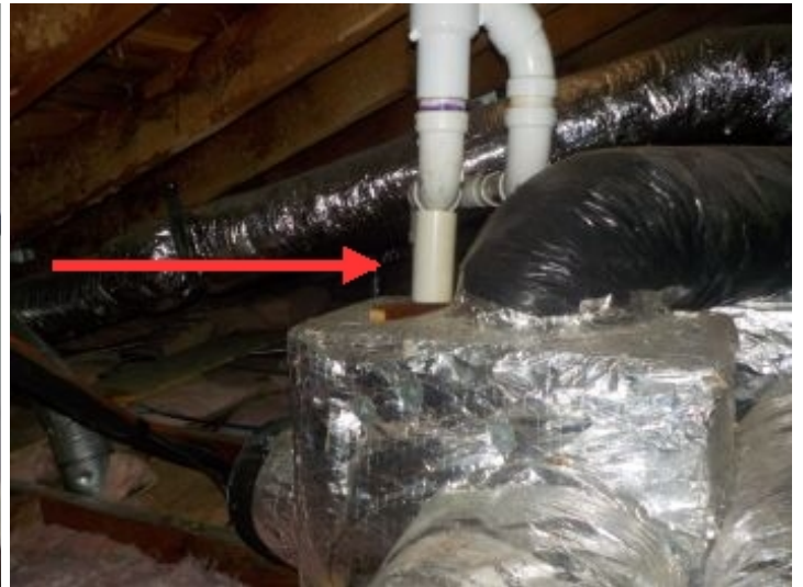
Attic, vents lines from the furnace, ( not the best practice)
