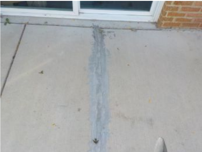
Patio, small hairline crack in the concrete.
