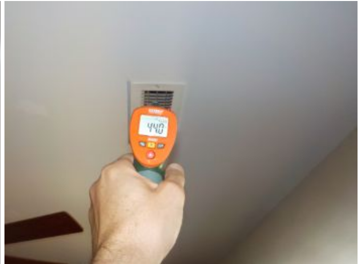
Cooling temp. OK
