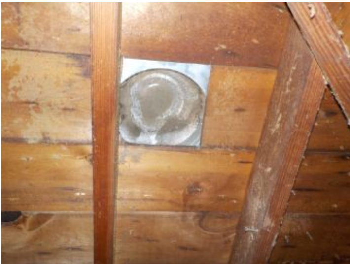
Attic vent dirty , should be cleaned on a regular basis.
