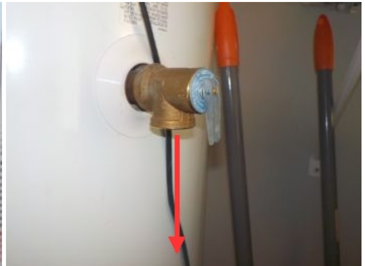
Pressure Relief Valve, pipe line should extend to the floor.
