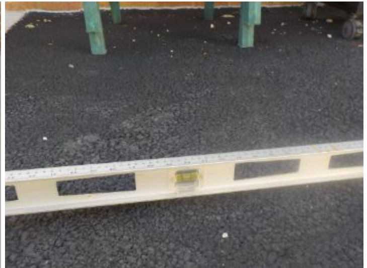
Patio, small crown that may lead to water pooling towards the home.
