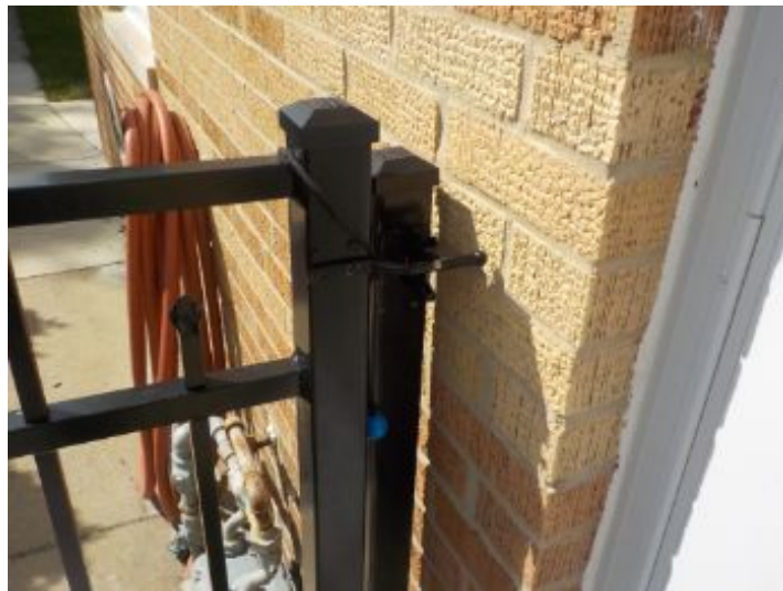
Gate does not close freely.
