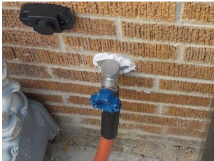
freeze protection bib installed on south of home.
