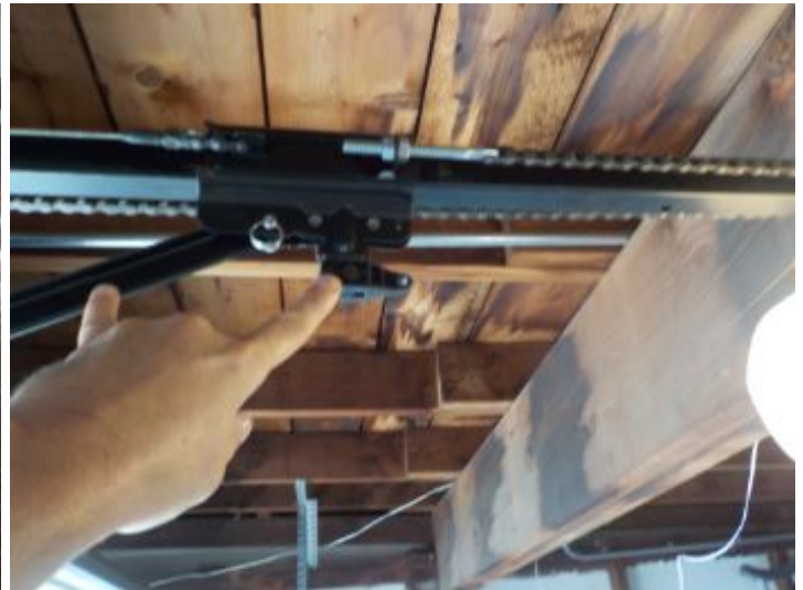
No manual string installed.
