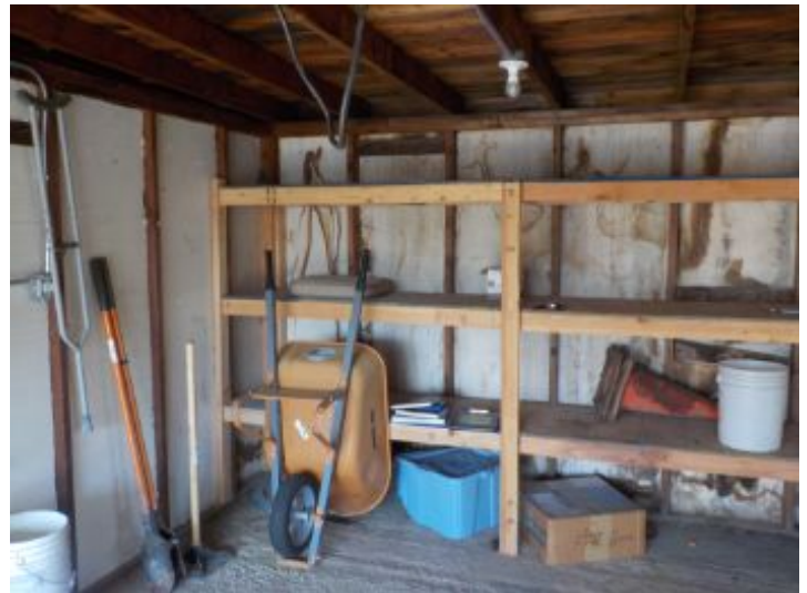
Garage, Evidence of moisture
